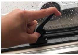
1 Press in the button on the bottom two handles and pull the lever upwards. The two side handles do not have buttons, so simply pull the levers to release.
